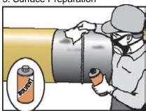
3. Insure that the surface is clean of grease, oil, salts, and other contaminants. If necessary, use Acetone, MEK or other suitable solvent. Perform cleaning when pipe is 3° C (5° F) above dew point.
